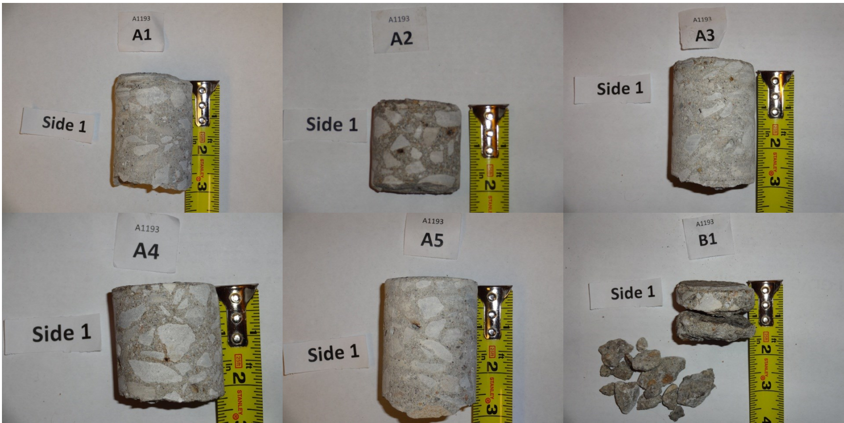
Figure 4-6 Cores Extracted From Bridge A1193
