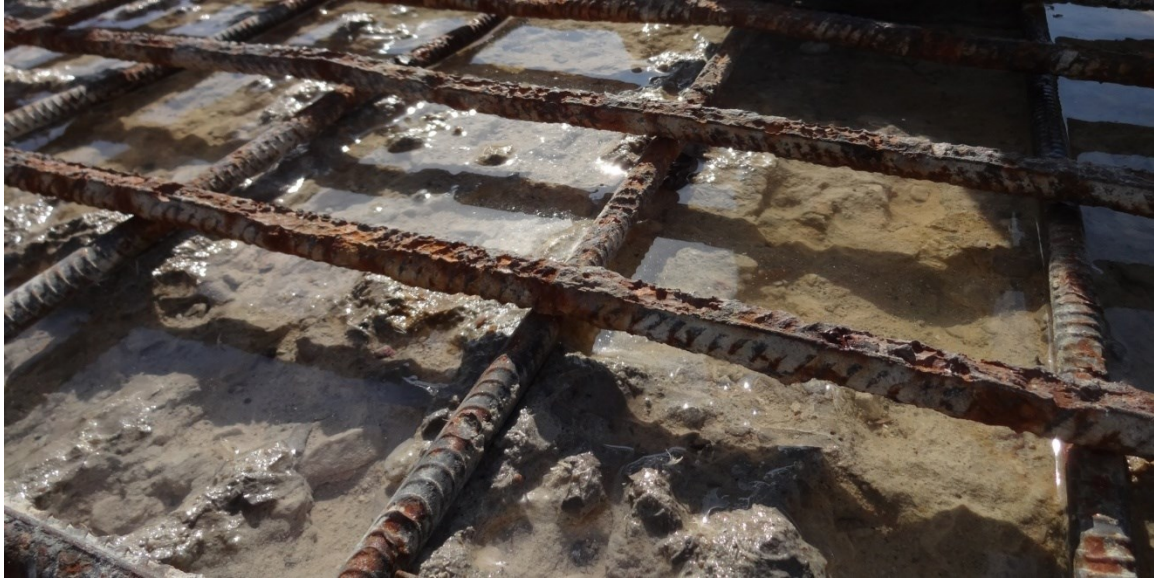
Figure 6-2 Corroded Rebar Exposed After Removal of Loose and Deteriorated Concrete by Hydro Demolition
