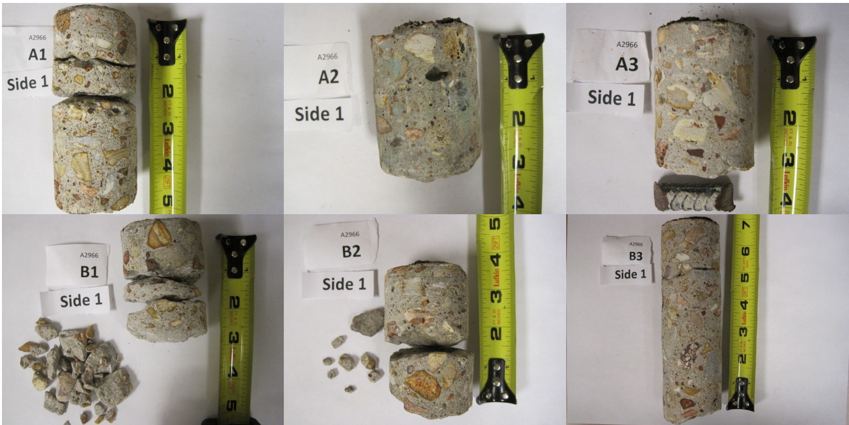
Figure 4-14 Cores Extracted From Bridge A2966
