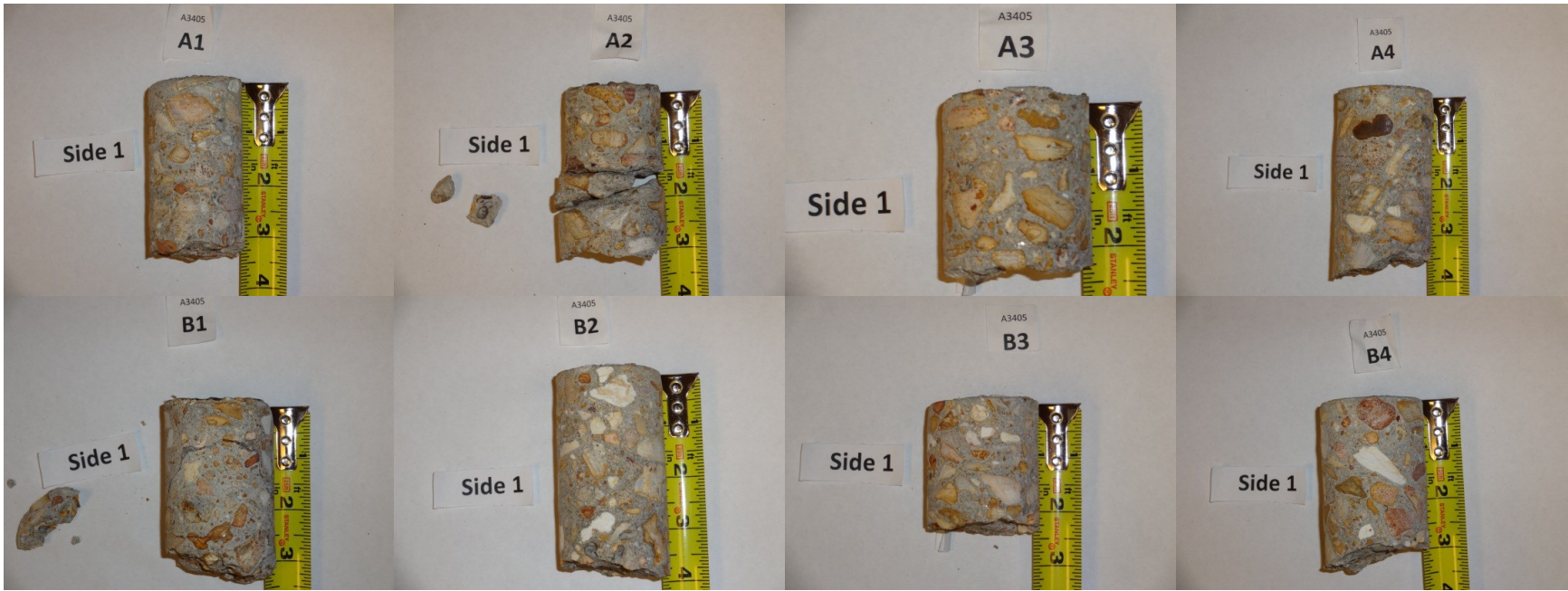
Figure 4-18 Cores Extracted From Bridge A3405
